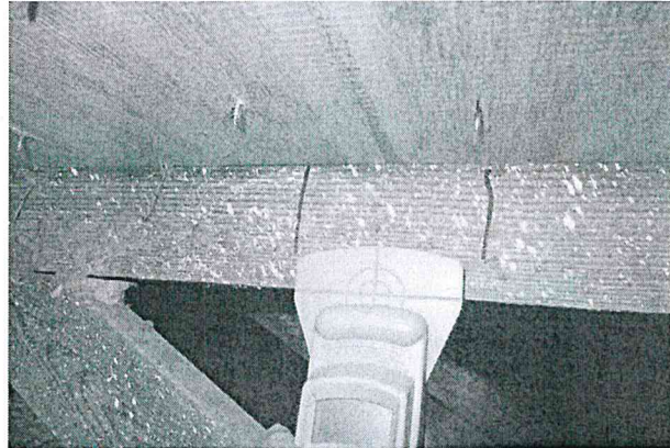
Single strap with 2 nails into the truss
